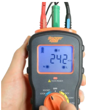
GOOD socket test and mains voltage
